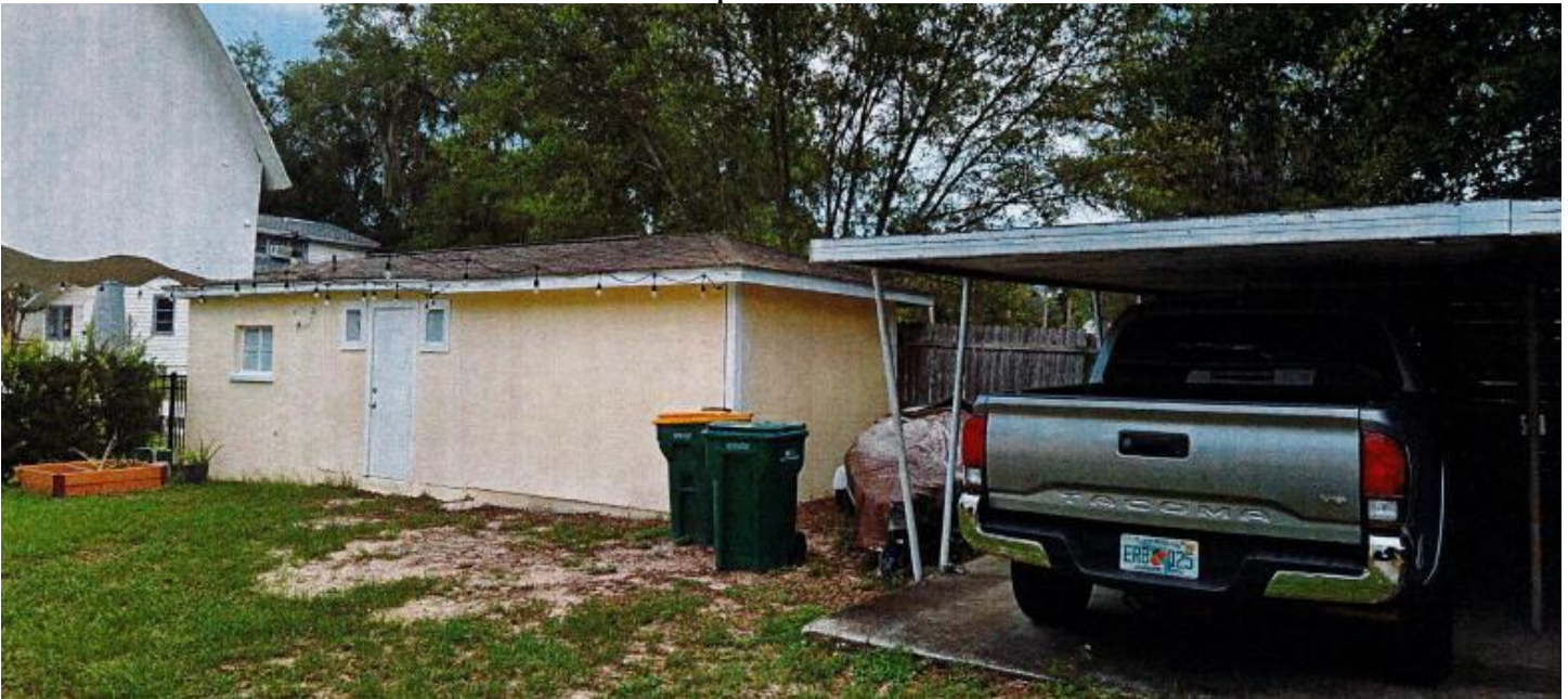
Structure Proposed for Demolition
