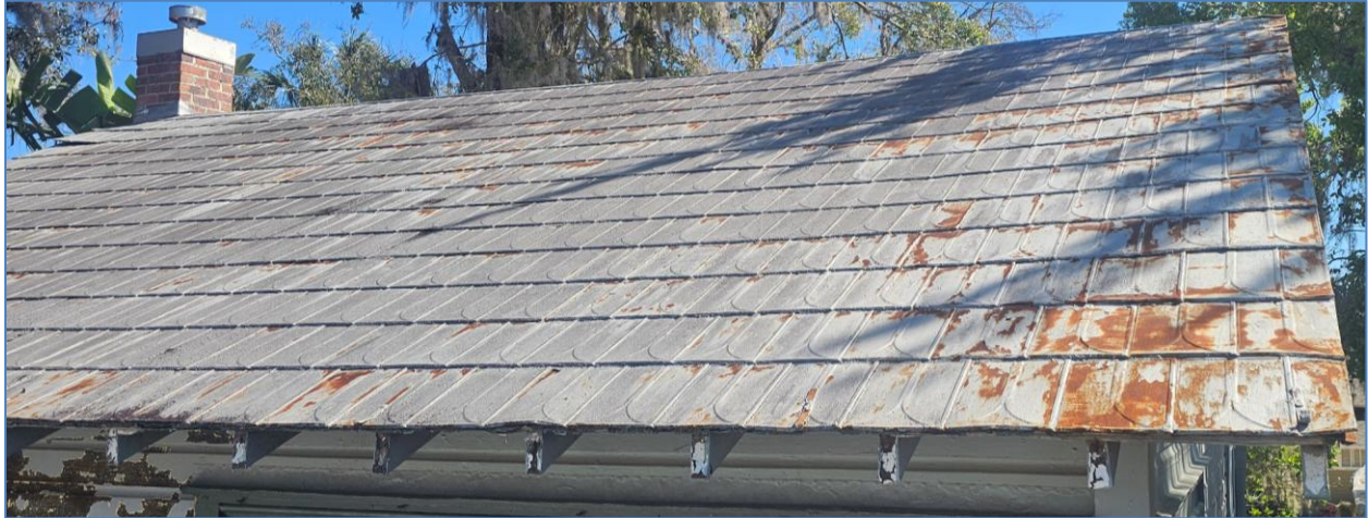
Existing Metal Shingle Roof
