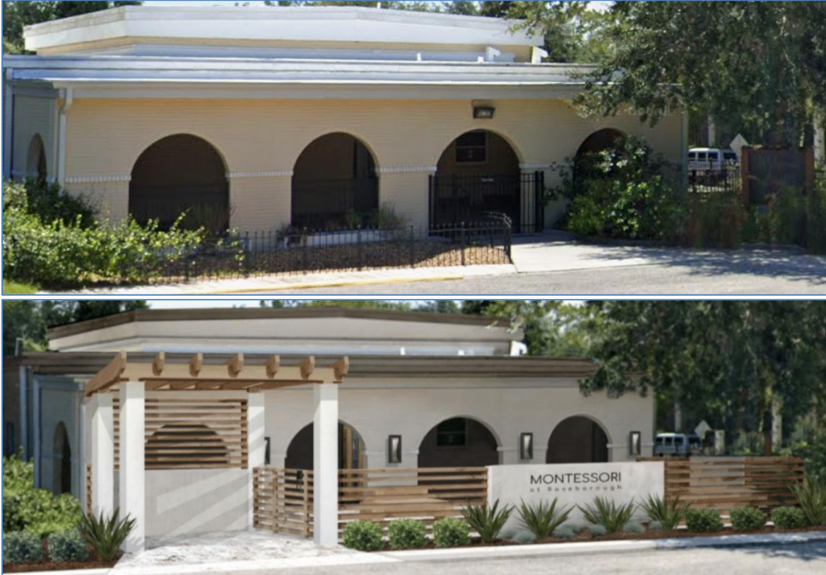
Existing Western Façade and Proposed Western façade depicting the proposed covered porch, open courtyard, entry pagoda, wood slat fencing, and stuccoed pillars & half wall.
