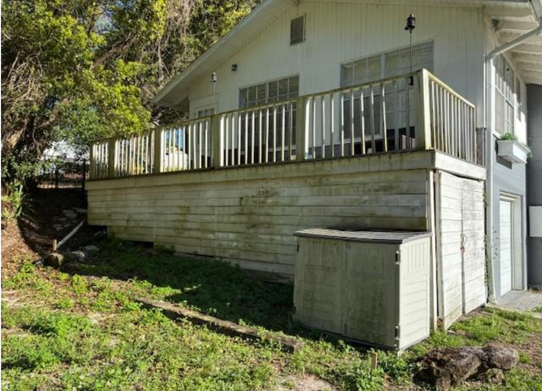
Current pictures of garage, shed, and deck.
