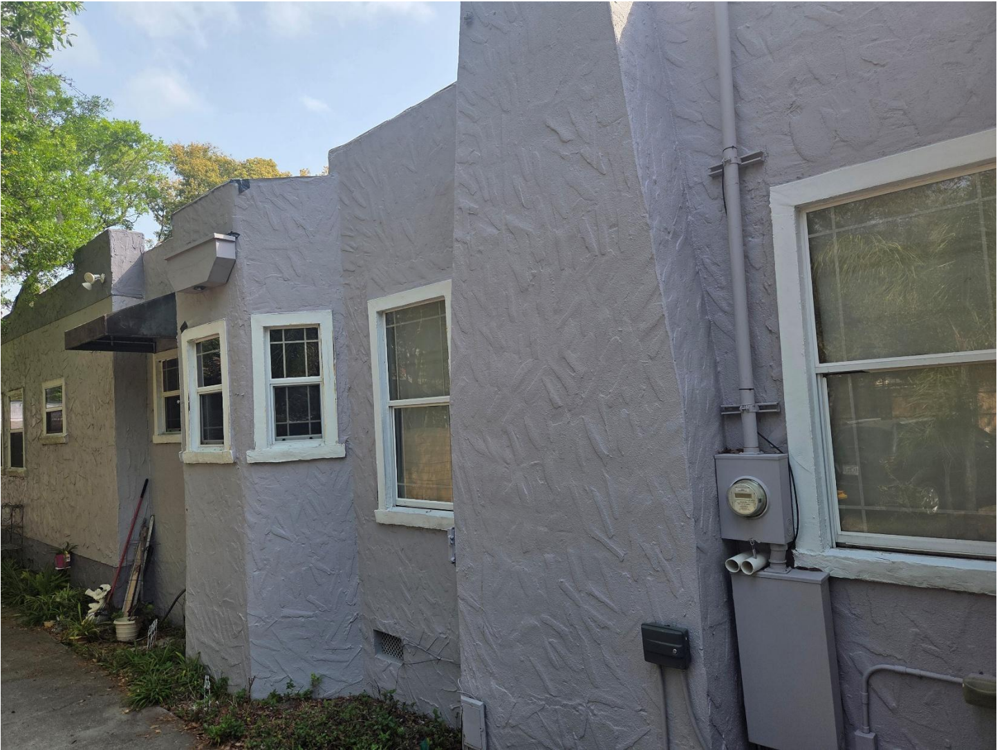
Western Side of House
