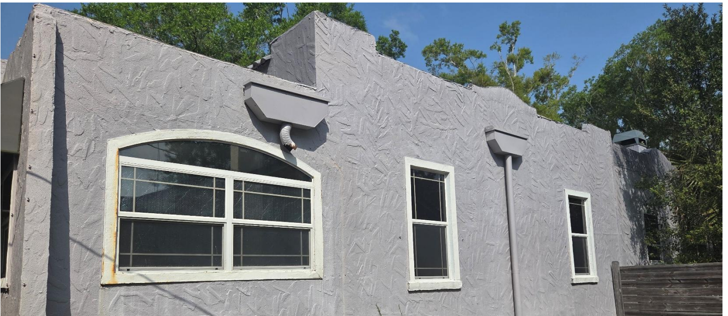
Eastern Side of House
