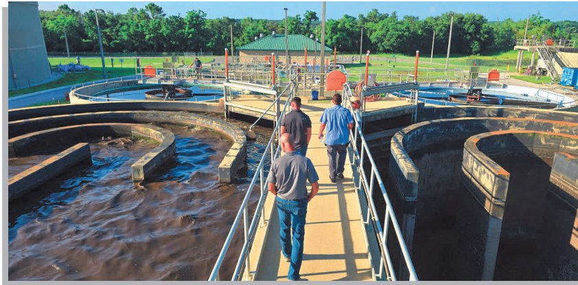
Eric Wagner, Tom Manning, Adam Corn, and Drew David Visited the WWTF #2 on July 21, 2025 with the City's Plant Staff.
