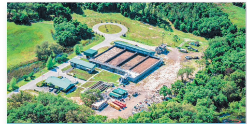
Turnpike WWTF City of Leesburg
