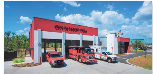
Fire Station #35 City of Mount Dora
