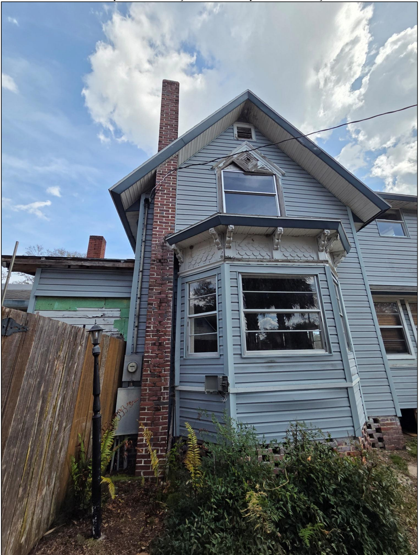
Chimney on Western Façade and Chimney on Northern Façade
