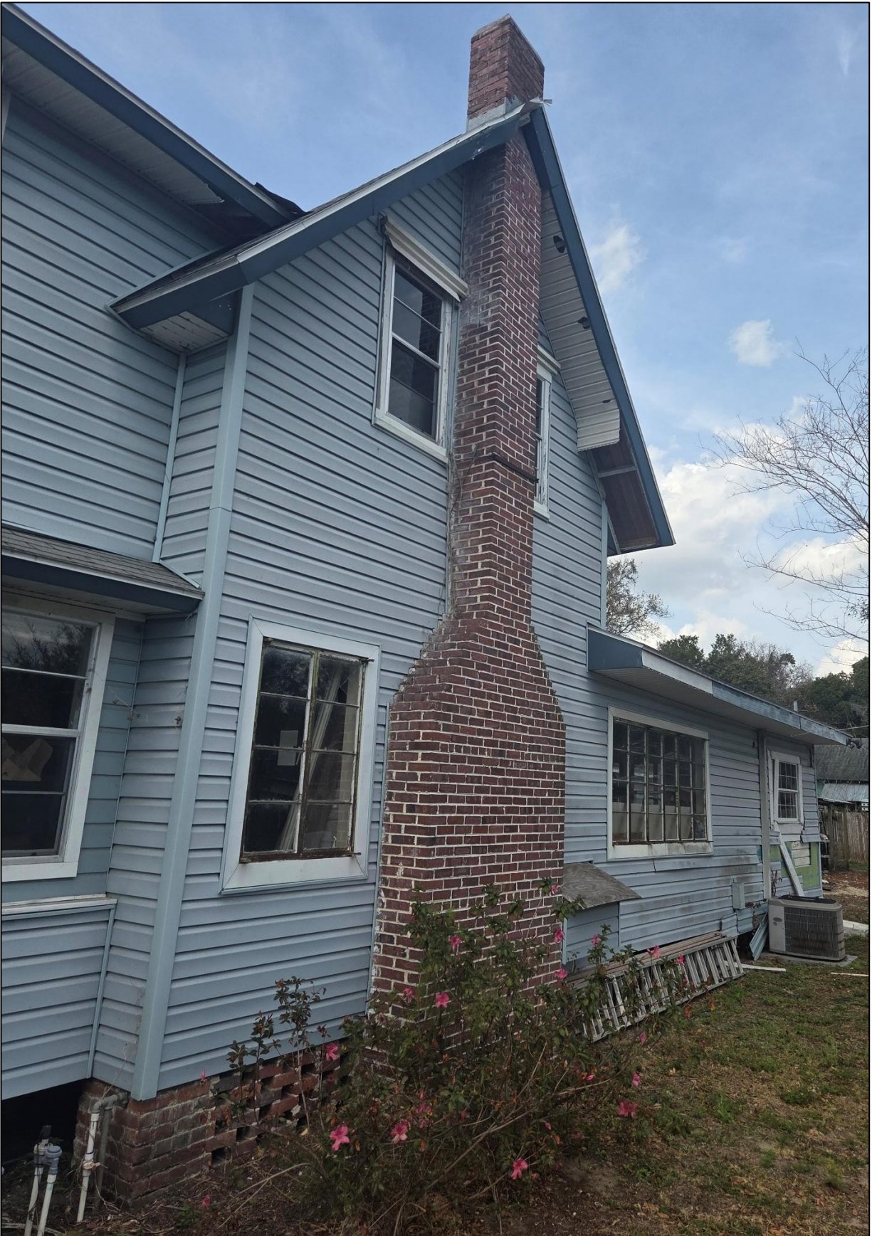
Chimney on Eastern Façade
