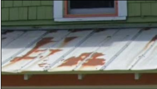
Existing Roof Panels
