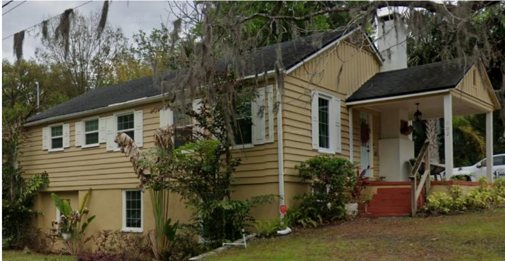
Existing Condition of the Western Façade
