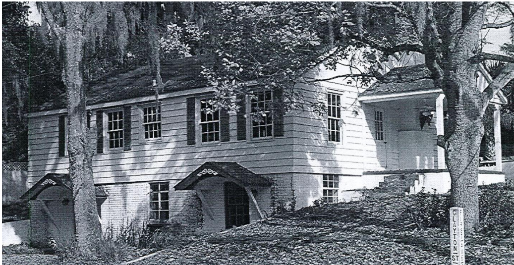
Western Façade of the residence from the 2008 Site File
