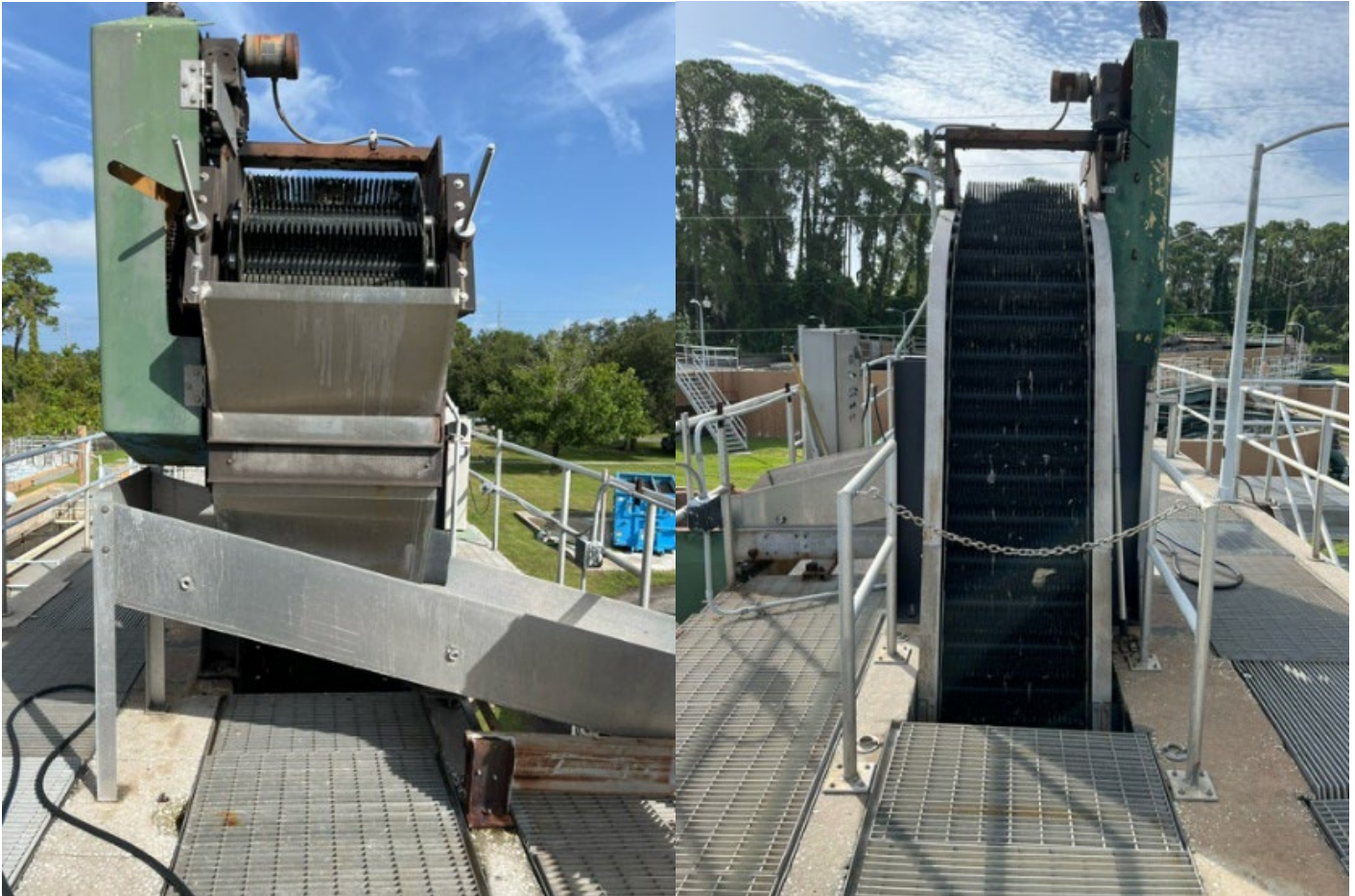
EXISTING EQUIPMENT AND SITE
