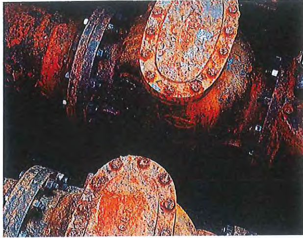
Figure 3 Check Valves
