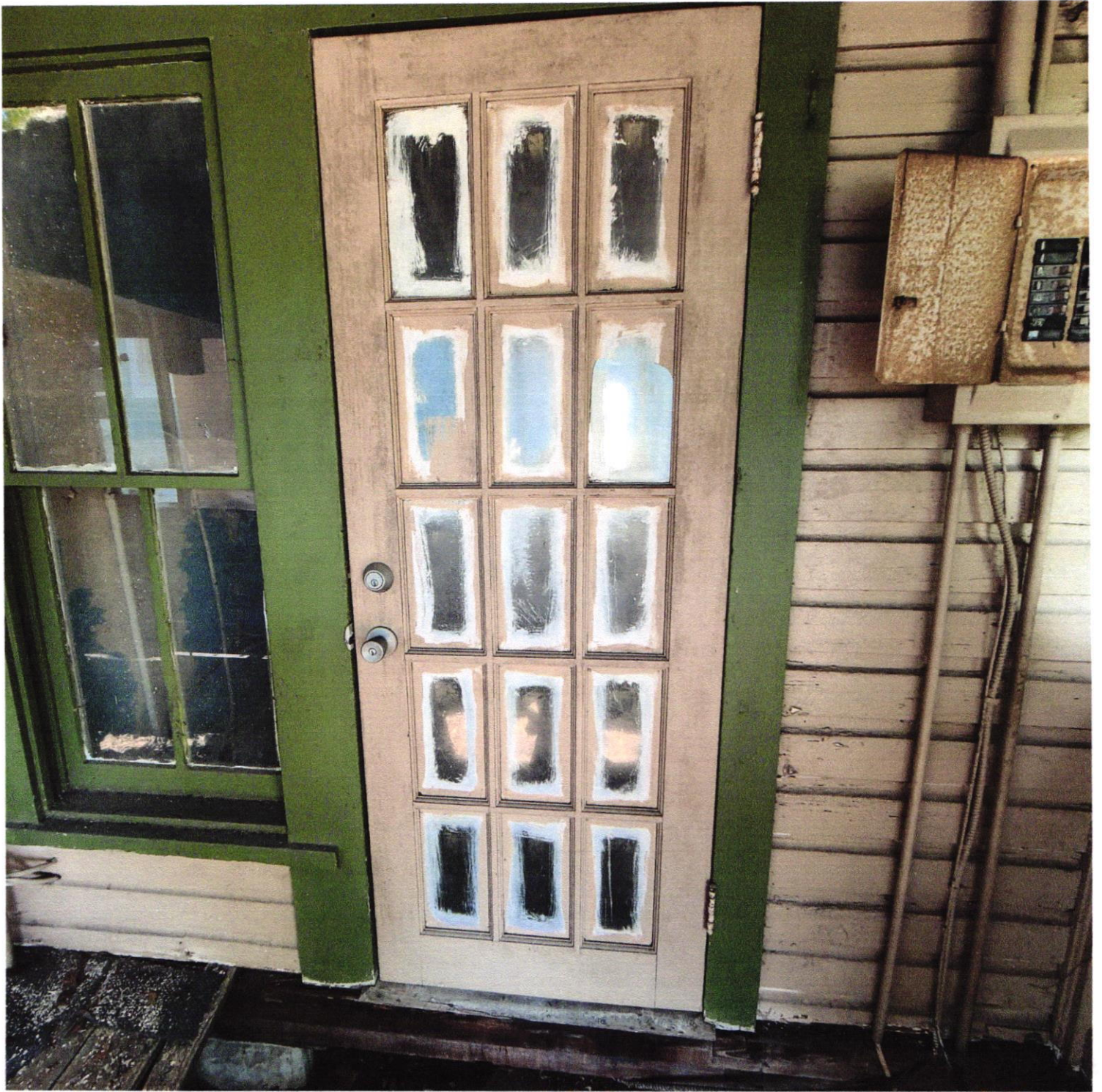
Existing door Replace w/ steel 15 lite door (new)
