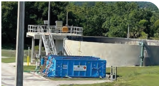
Halff Site Visit | May 2024
