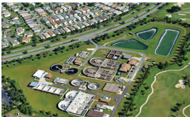
Troy Mitchell Experience | Central Sumter Utility Wastewater Treatment Plant
