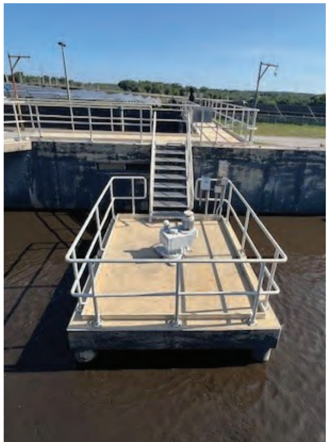
Halff Site Visit | May 2024
