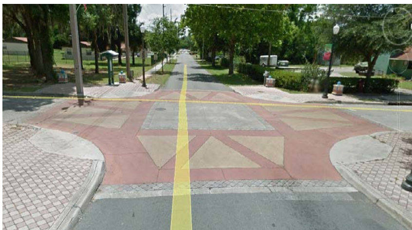
Figure 3: Grandview St and Lincoln Ave intersection
