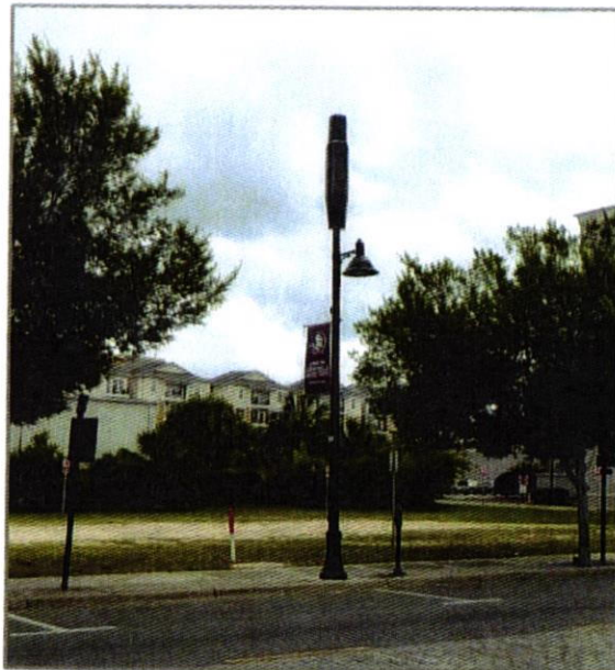
Tallahassee Decorative Light Node/Pole
