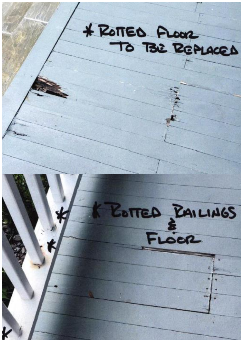
Current Wood Porch
