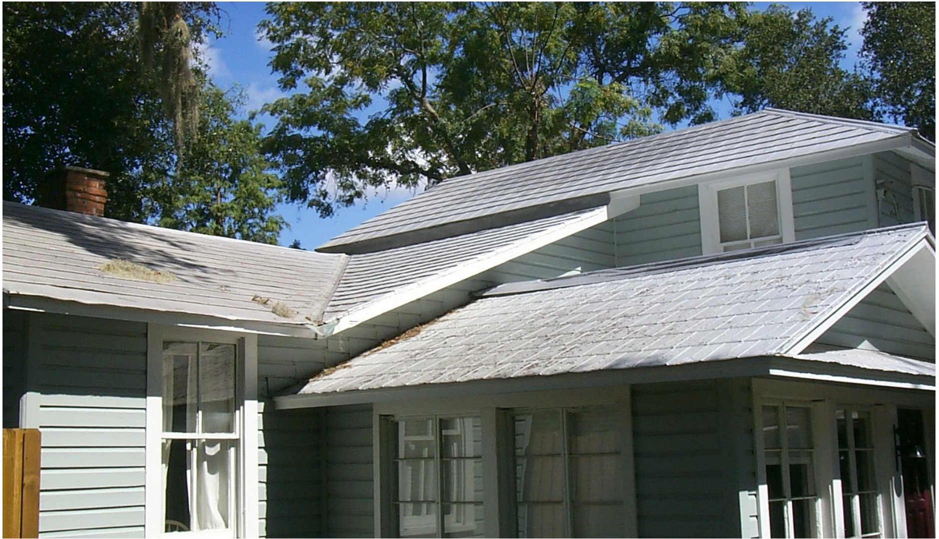
Photo 1 – View of left (west) side of roof area.
