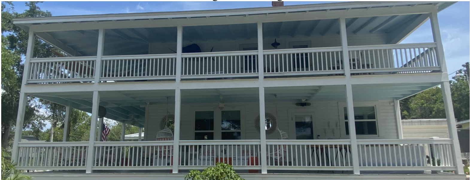
Existing Wood Railings:
