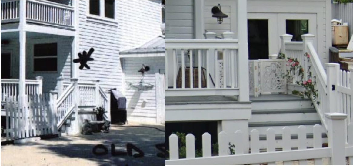
Rear Wood Steps
