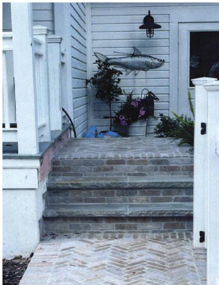
Rear Concrete Steps
