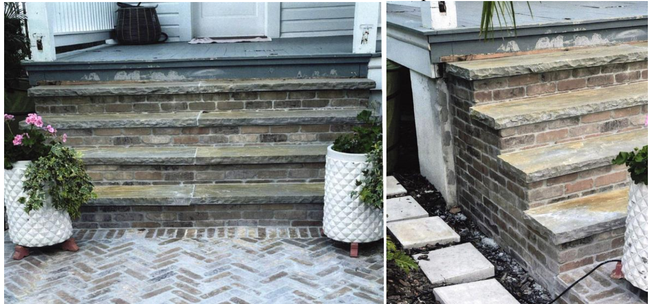
Front Concrete Steps
