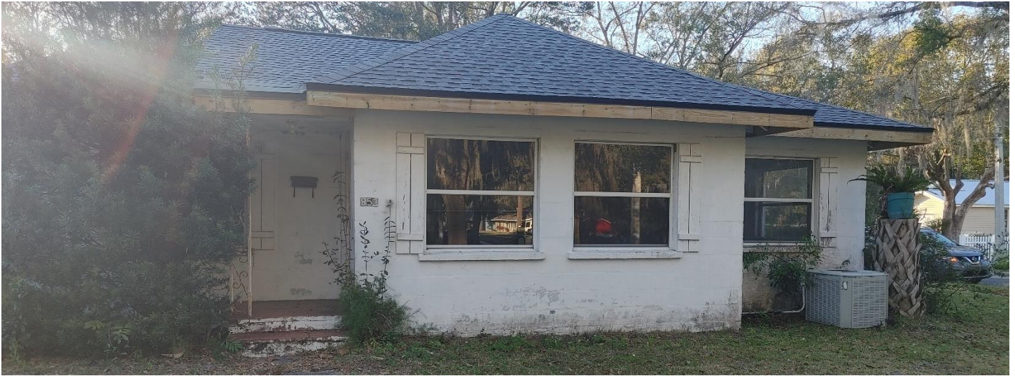
Eastern Elevation, Fronting Clayton Street
