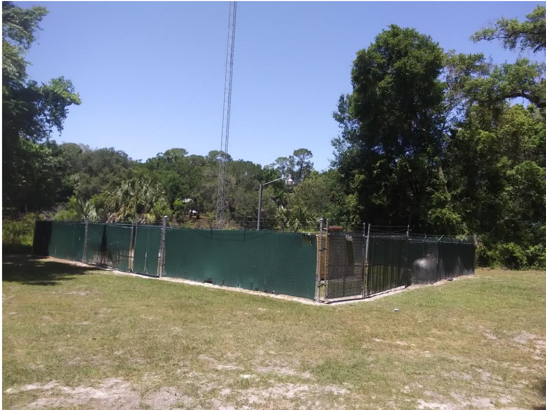
19) City of Mt Dora Forest Preserve – Water Treatment Substation along west side of Lake John
