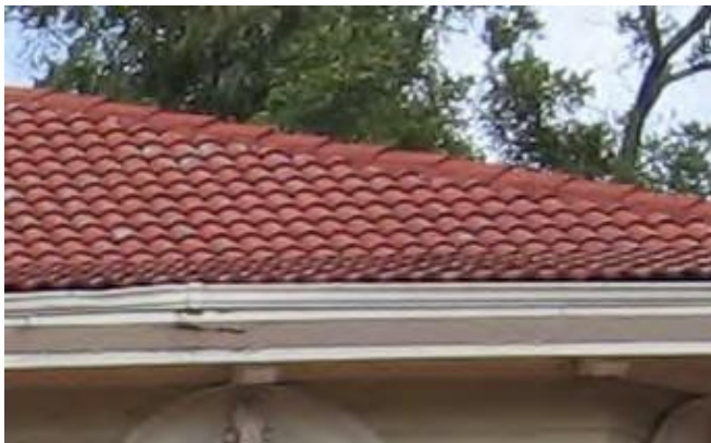
Retain and preserve original roof materials such as fired clay tile. (315 Alachua Avenue)
