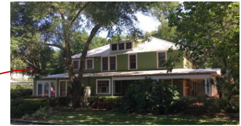
950 North McDonald Street - 10th Ave. View
