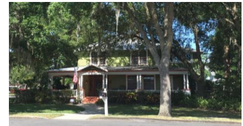
950 North McDonald Street - McDonald Street View
