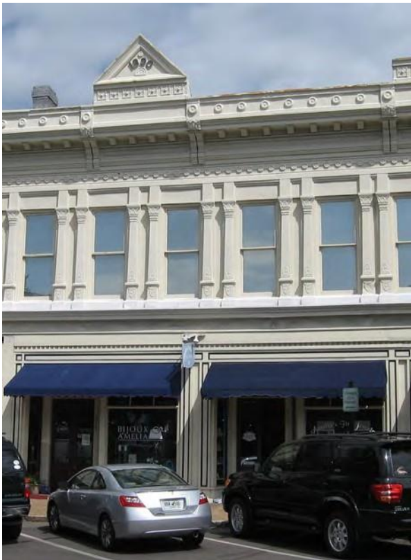
Metal façade at 313-319 Centre Street.
