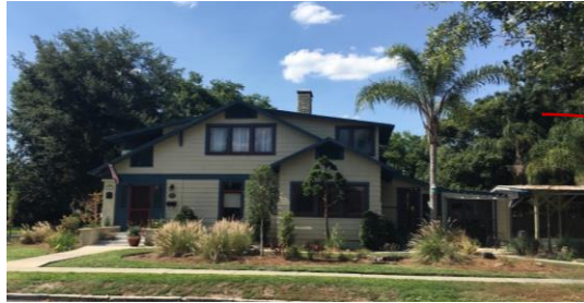
315 Helen Street - 10th Avenue View
